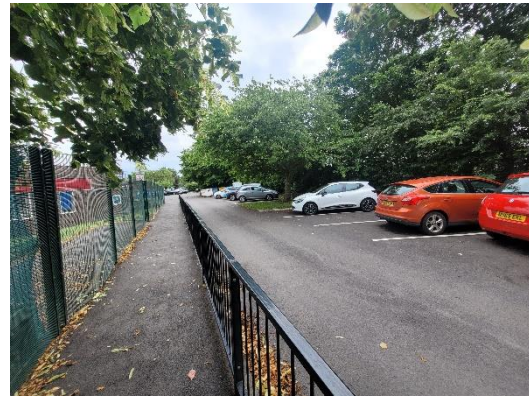
Resurfacing & Additional Parking Bays.
